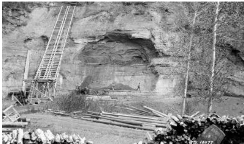
Figure 9.11 Oil sands were first exploited as a ready-made source of asphalt. Mining "tar sands" near Waterways, AB, in 1925.
