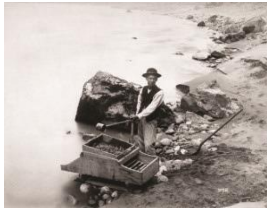
Figure 9.31 Chinese miners introduced machinery like this “rocker” on the Fraser River ca. 1875.
