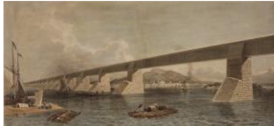
Figure 10.7a The Victoria Bridge was part of the Grand Trunk Railway's infrastructure and, at the time of its completion in 1857, the longest span on Earth.
